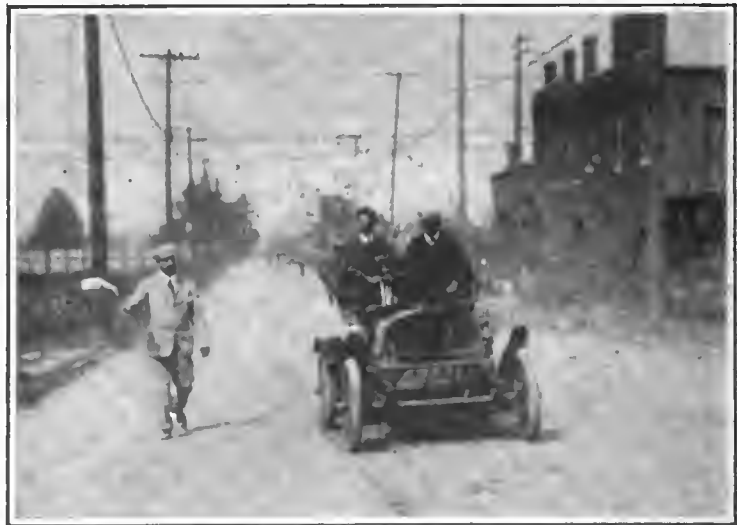
DIRECTING FRANKLIN CAR THROUGH EAST ST. LOUIS TO BRIDGE.
